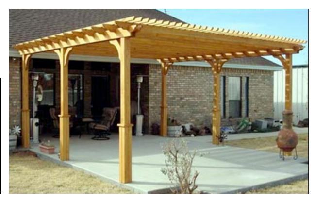
This picture illustrates the six support posts and overhead style crisscross pattern. The first row of rafters are 2"x6" and 8" off center. The material for the top row will be 2x6's ripped into thirds and placed 2" off center. Instead of notching, galvanized T-brackets will be used which eliminates toe-nailing. As in this photo, the ends of the rafters and top rails will also be decoratively cut for esthetic purposes.
